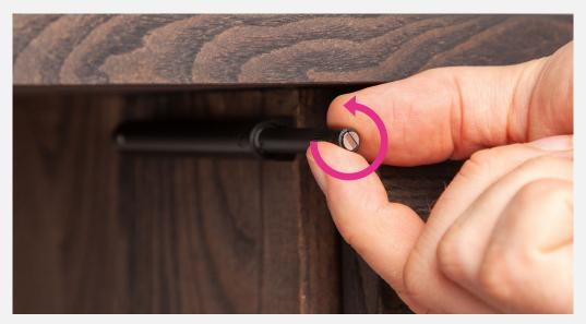
**3:** On the opposite side of the door, the regulating pin can also be adjusted in or out on the push mechanism to achieve the desired result. *NB: Never screw the regulating pin fully in, as the push mechanism does not work then and the door may be difficult to open again!*
