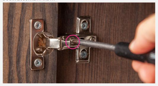
With this screw the doors can be adjusted in the width. Close the door and check if the distance fits - repeat the adjustment until the desired result is achieved.
